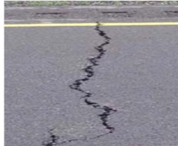
Transverse Cracks
