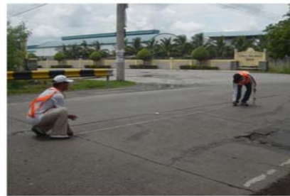
3. Measure length of affected area
