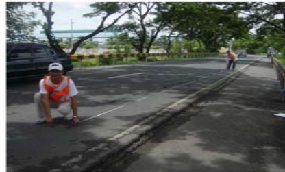
3. Measure length of failure
